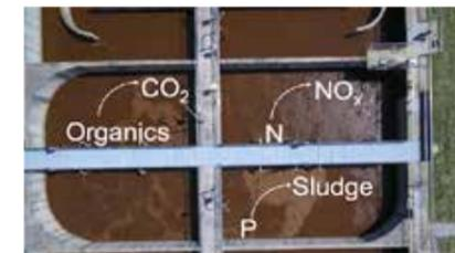
Figure 1. Scheme of conventional activated sludge wastewater treatment plant
